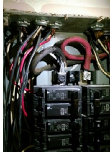
One of Outside panels... notice the wire melted at the top of fuses.
