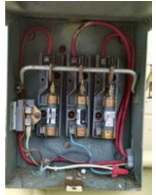
One of Outside panels... notice the wire melted at the top of fuses.
